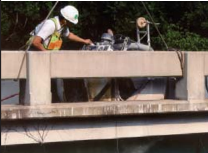
As the bridge rails are removed, a new bridge deck is being constructed between the two existing ones to provide one seamless bridge with northbound and southbound lanes.
