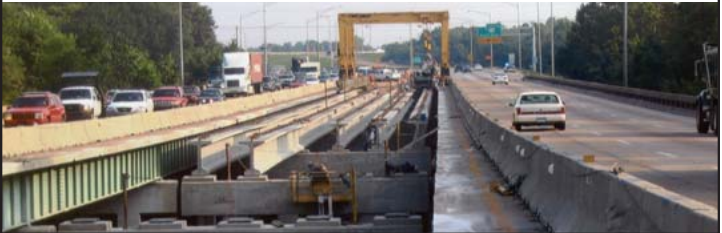
As the bridge rails are removed, a new bridge deck is being constructed between the two existing ones to provide one seamless bridge with northbound and southbound lanes.
