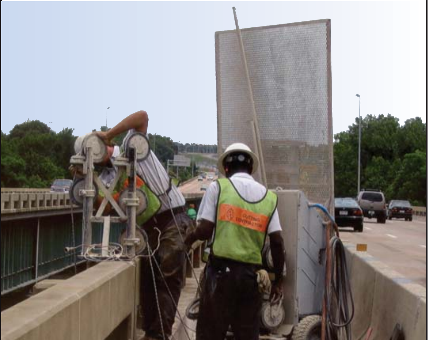
ABC Cutting operators set up the wire saw unit behind a protective screen.
