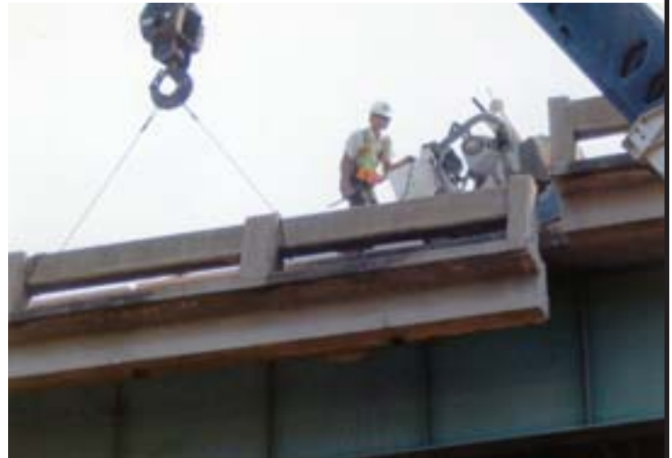
As the bridge rails are removed, a new bridge deck is being constructed between the two existing ones to provide one seamless bridge with northbound and southbound lanes.
